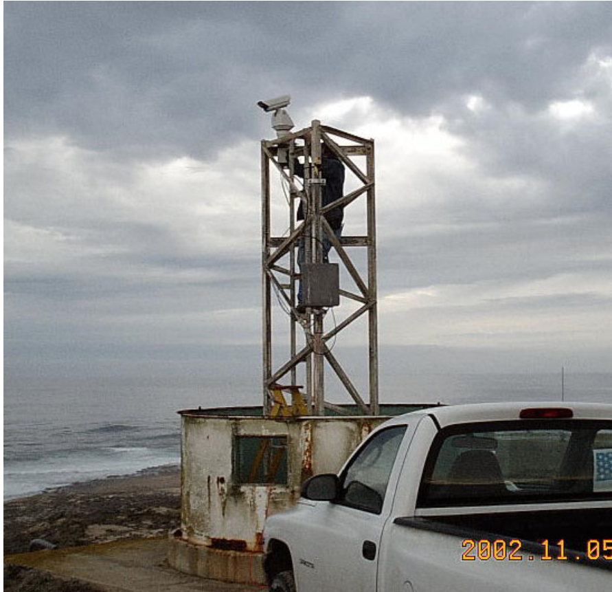
FIGURE 3.2. View of the permanent fixed video camera at Building 809. This camera can be remotely zoomed, tilted, and panned, but was non-operational during the present monitoring period. (Photograph by U.S. Navy)
