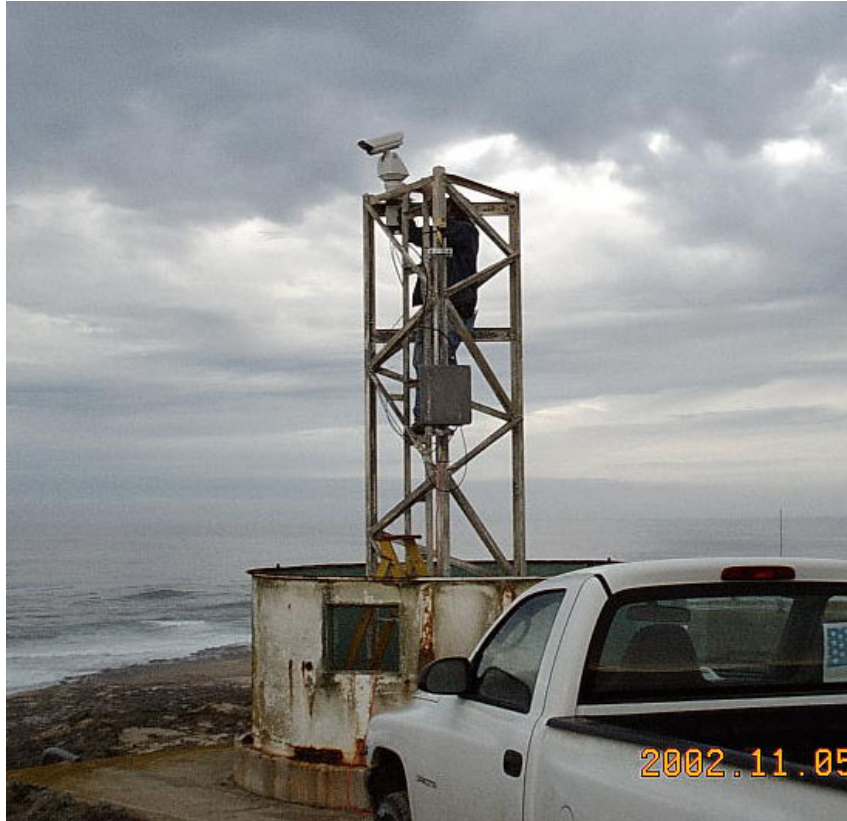
FIGURE 3.1. View of the permanent fixed video camera at Building 809. This camera can be remotely zoomed, tilted, and panned. (Photograph by U.S. Navy).
