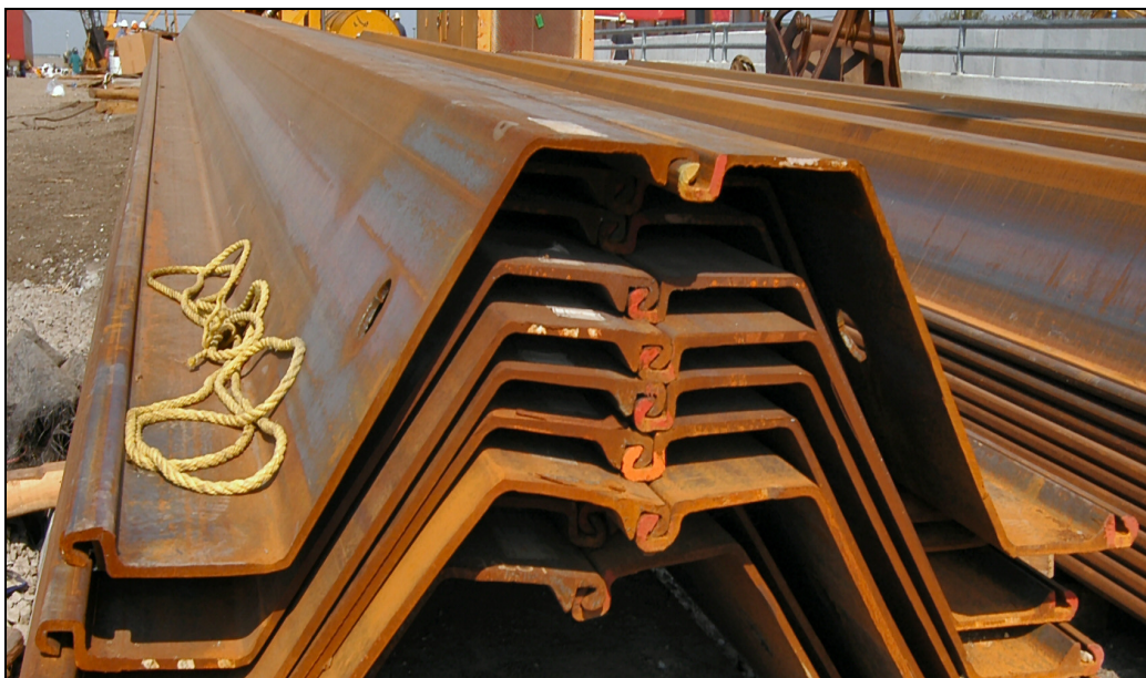
Figure 1: One-foot piles that get interlocked during pile driving events.
